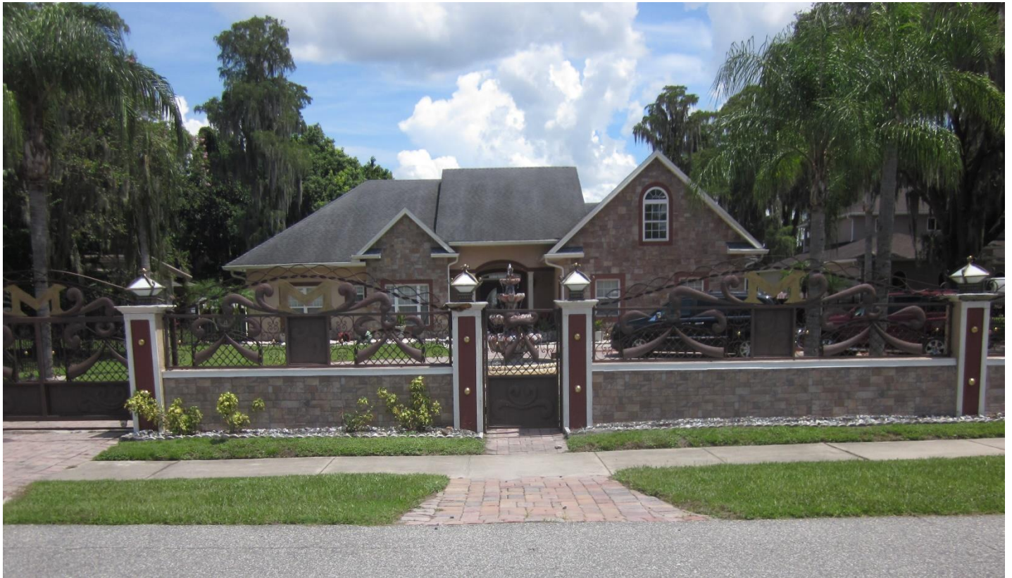
6.3 ft. high columns with a 5.4 ft. separation in lieu of 10 ft.
