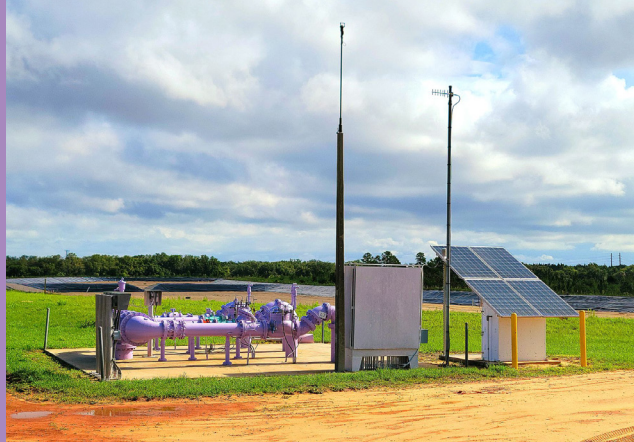
Solar-powered reclaimed water meter assembly at Water Conserv II
