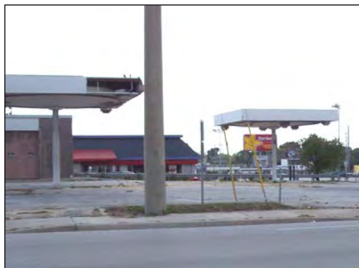
Figure 6: Image of vacant gas station at the Pine Hills/Silver Star intersection
